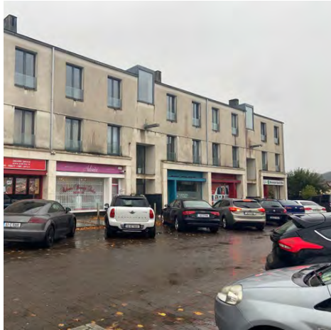
Newer development in the town feels out of sync with the town centre core, in terms of scale and massing, roofline design, and condition.
