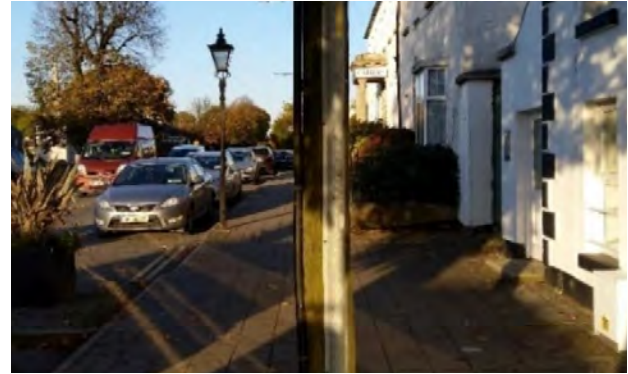
Figure 38 Example of poorly placed service poles
