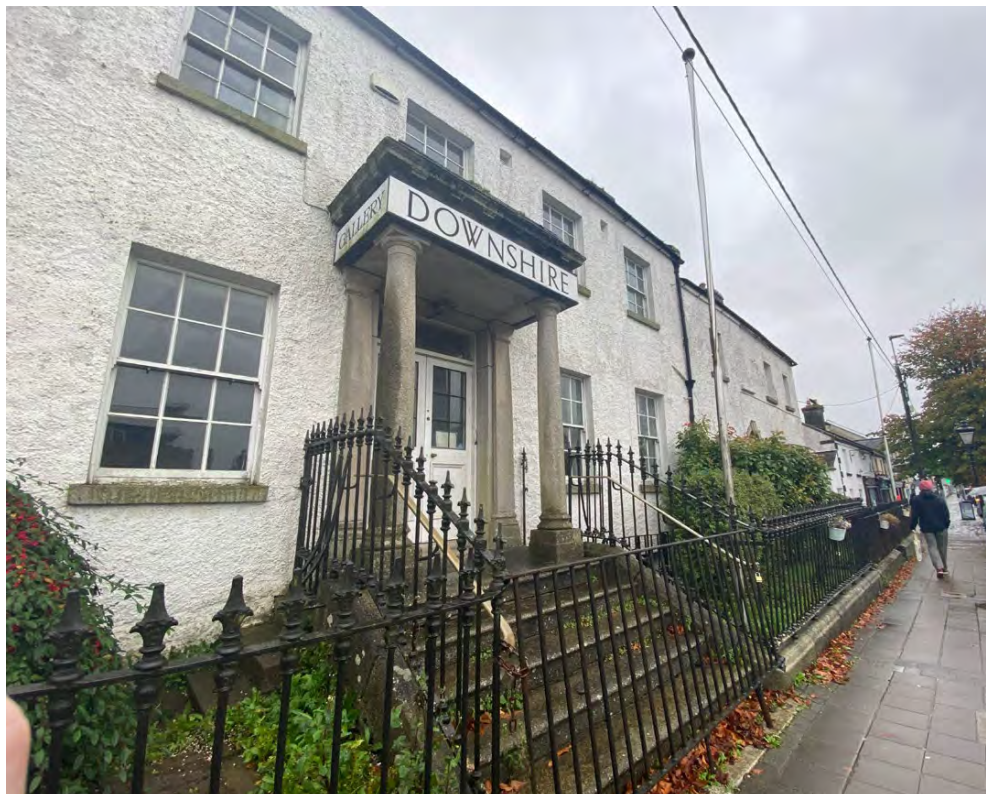
The prominently location, and vacant, former Downshire Hotel occupies a prime town centre site with generous backlands.
