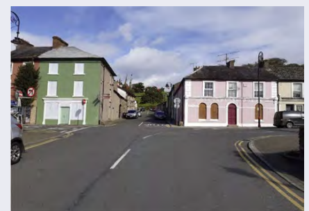
Refurbished residential accommodation in Cappoquin
