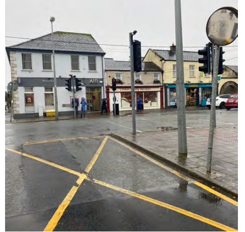
Narrow pedestrian crossing along Main Street
