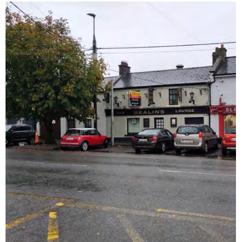
Overhead electrical cabling is a constraint to retention of existing street trees and planning for more.
