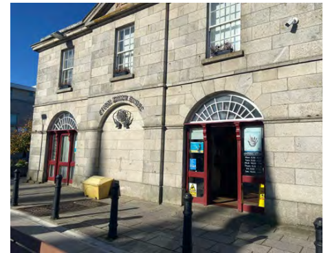
Main Street is enhanced by significant buildings such as Market House (now Credit Union), a Protected Structure. Details such as the materials, door cases, windows, particularly where these are original or older and the carriage arches at intervals along the street make a significant contribution to sense of place.
